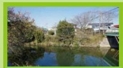
Remains of Eidaibashi Bridge It was a bridge on the Bonotsu Kaido.
