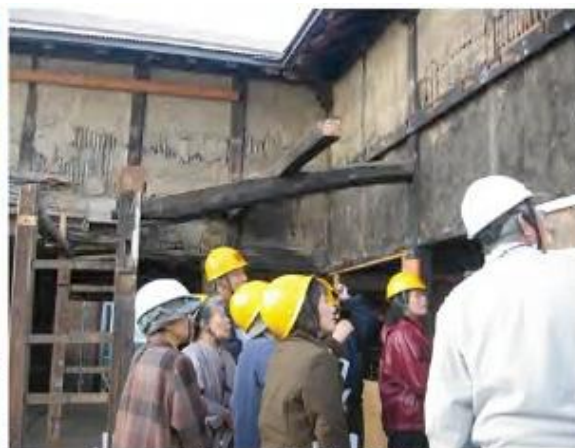
Restoration work tour
