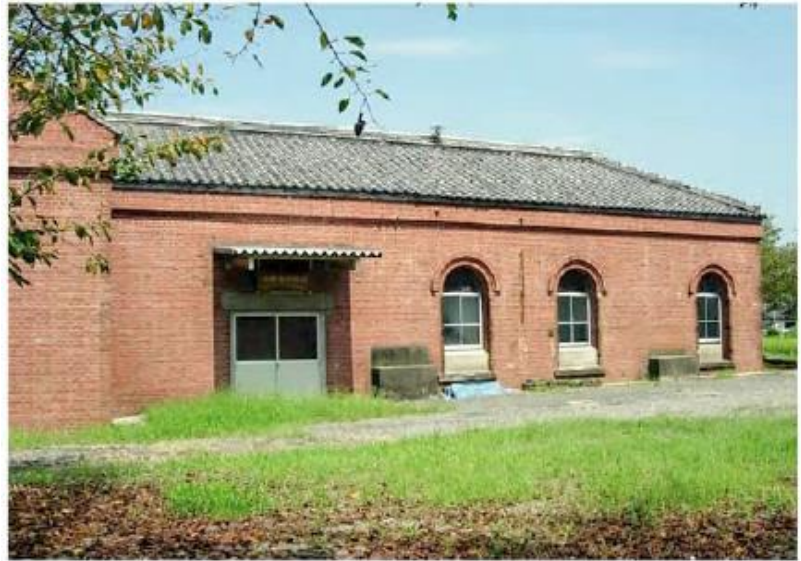
Former Miidera Pump Station
