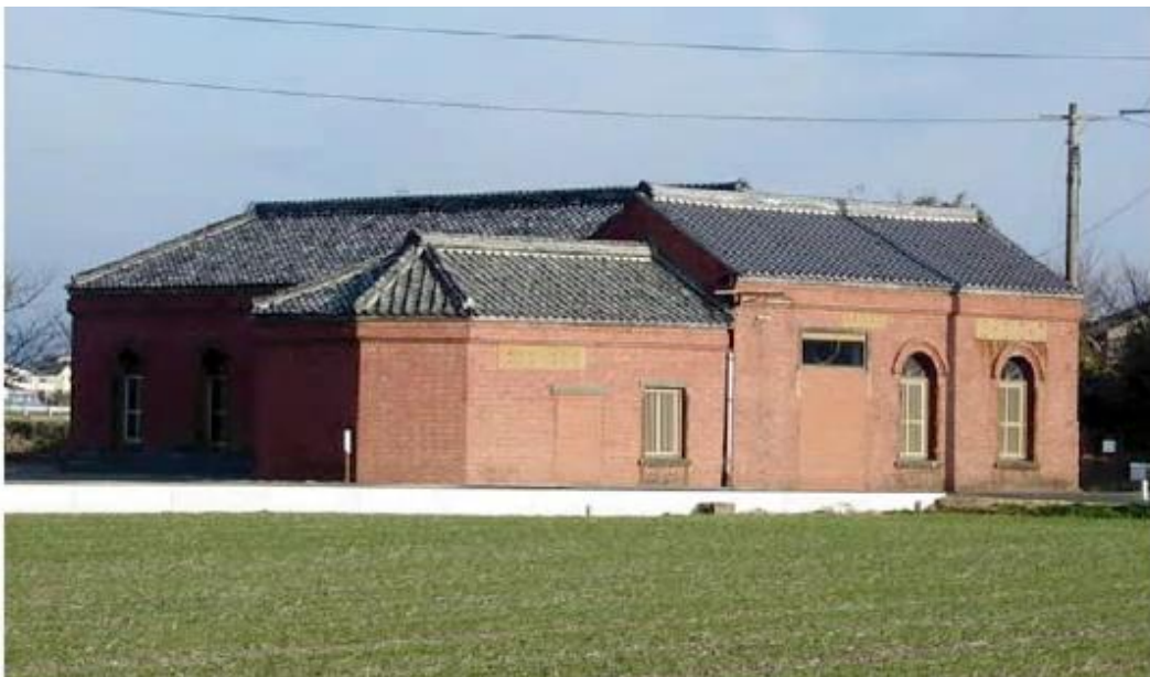
Former Miidera Pump Station and Electricity Substation
