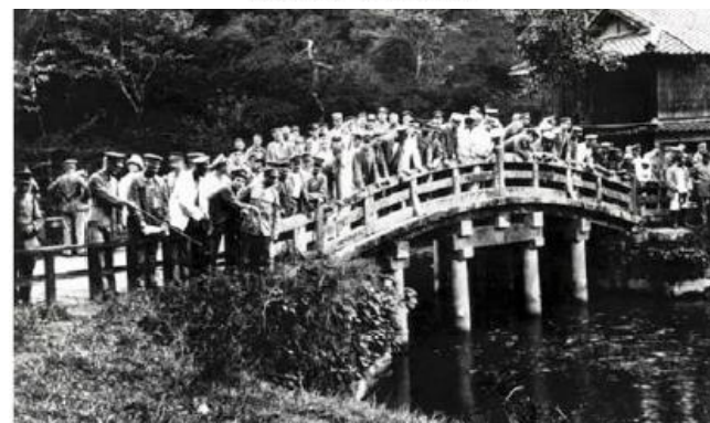
On the Mitarai Bridge
